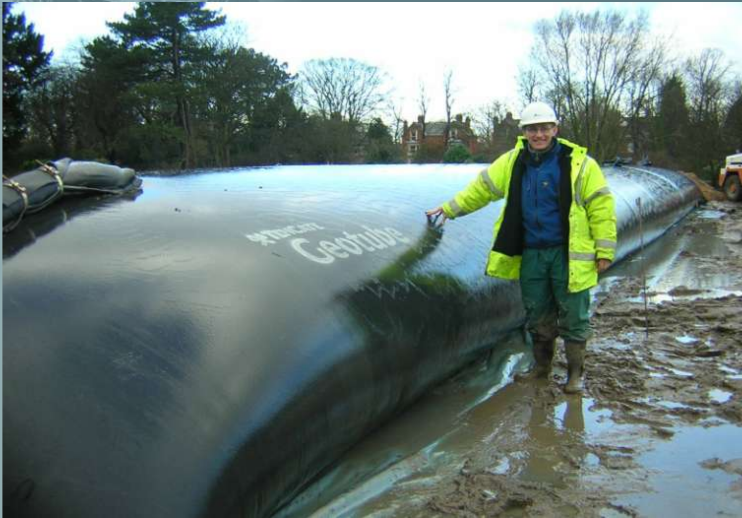
Silt removal from discharge water using geotextile bags
